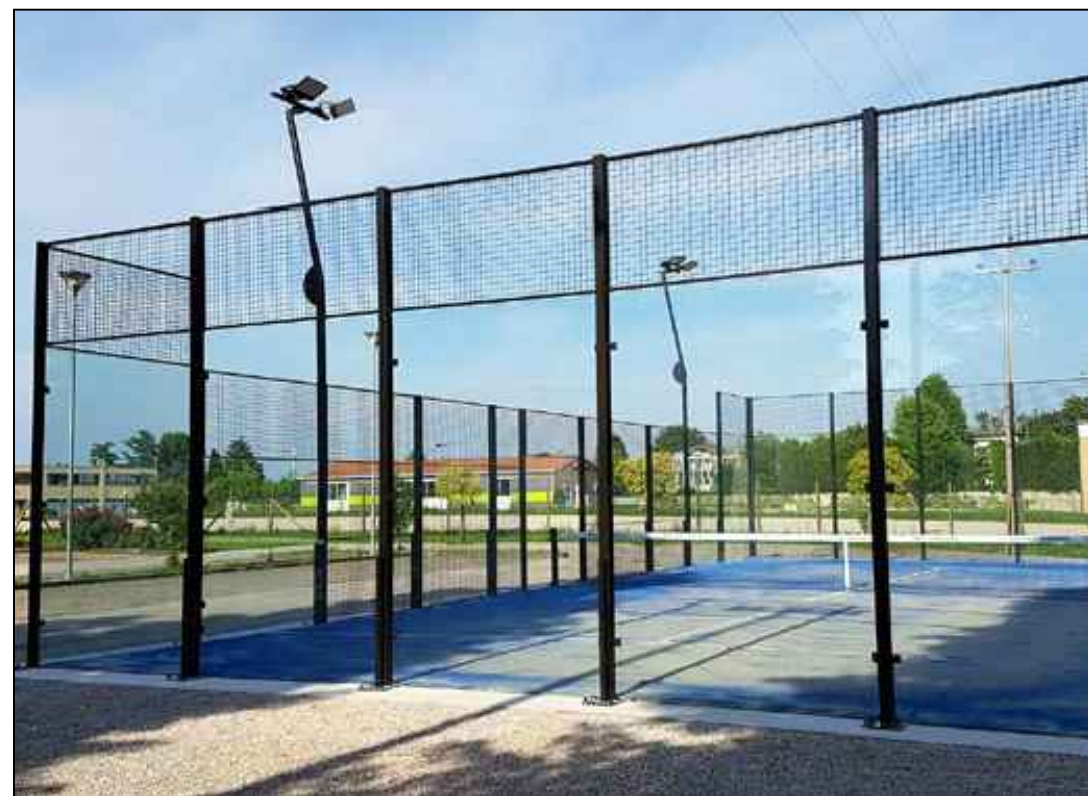
Padel Court Fencing
